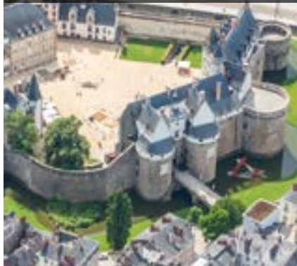
The courtyard of the Castle Soiree in a 360° architectural theatre
